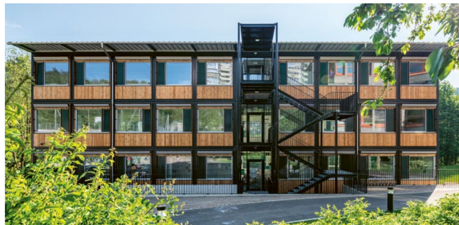
ZM10 school pavilion, Sihlweid Zurich
