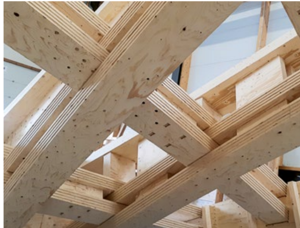
The mockup established trust. For the client, the suppliers and within our own project and assembly teams. Well visible: the five layers of beams, each consisting of five LVL lamellas. The shear connectors that join the layers of beams can also be seen.
